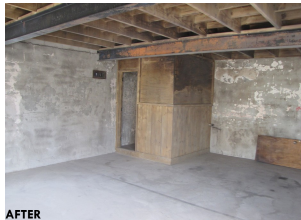
Smoke and soot damage removed for recoating
