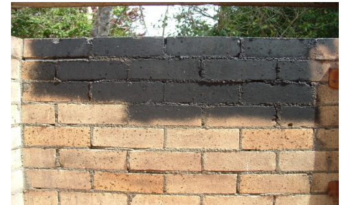
Removal of smoke damage to a brick wall
